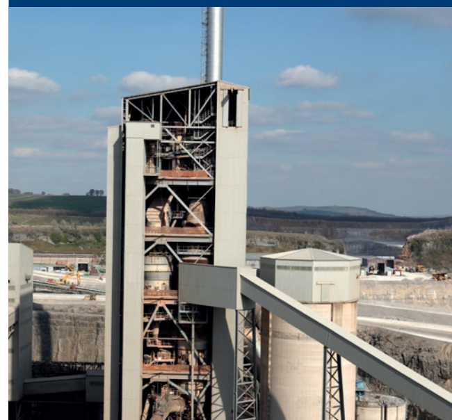
Figure 9: Modern plant cyclone suspension preheater tower at Tunstead.
