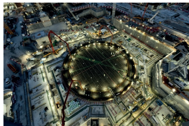
Figure 12: Hinkley Point C construction hit the record books in 2019 with the longest continuous pour of concrete (9,000 cubic metres over five days).
