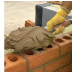
Mortar – a basic building material needing cement
