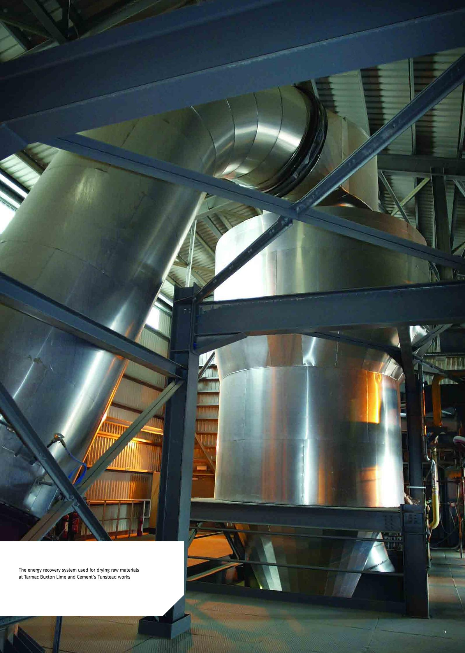
The energy recovery system used for drying raw materials at Tarmac Buxton Lime and Cement's Tunstead works
