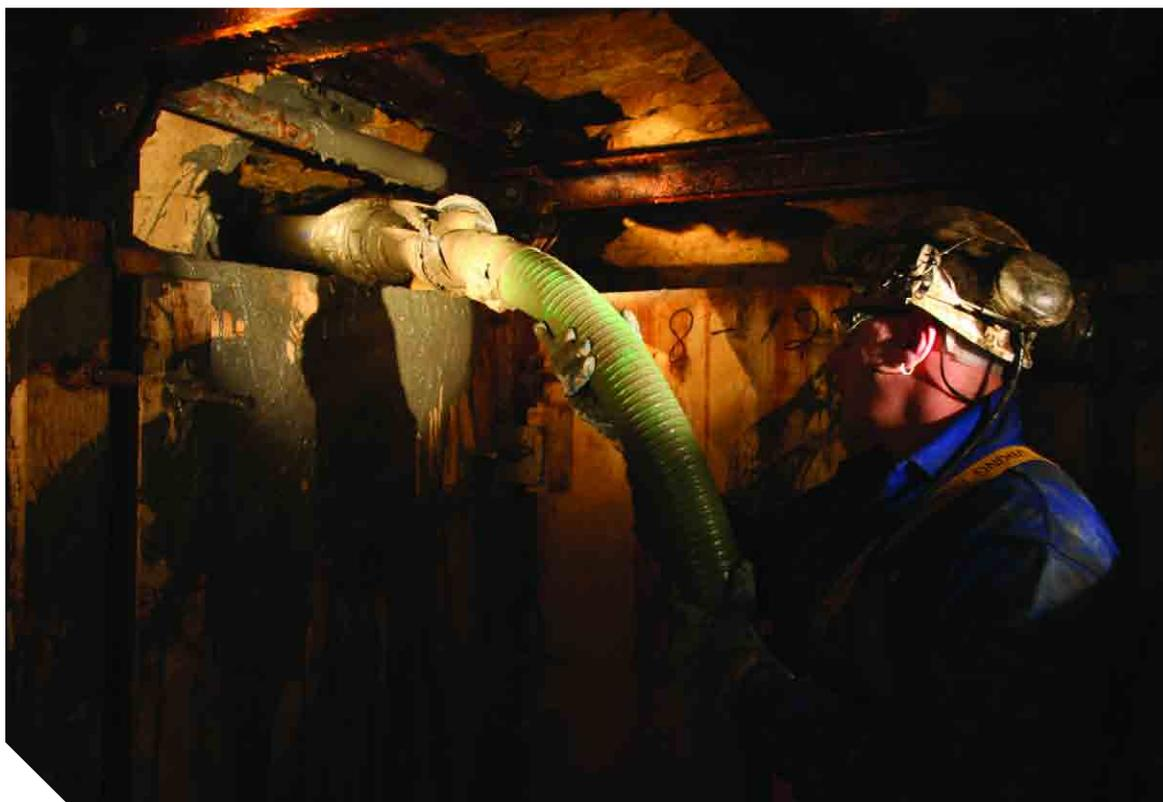
Cement from CEMEX UK's Rugby plant is being used in pumped concrete, which is pumped into old mine workings beneath the village of Combe Down near Bath to stabilise conditions
