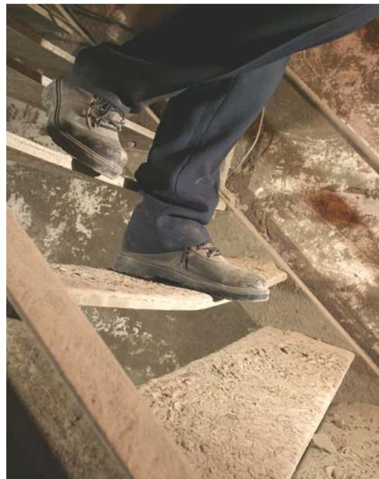
Worn stair treads lead to slips, trips and falls.
